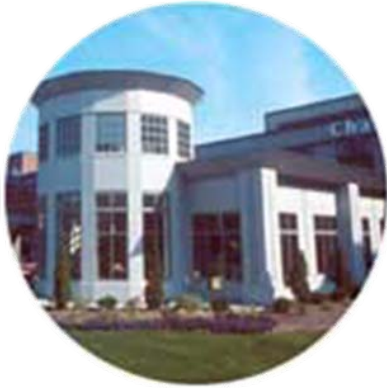
Charlton Memorial Hospital Fall River
